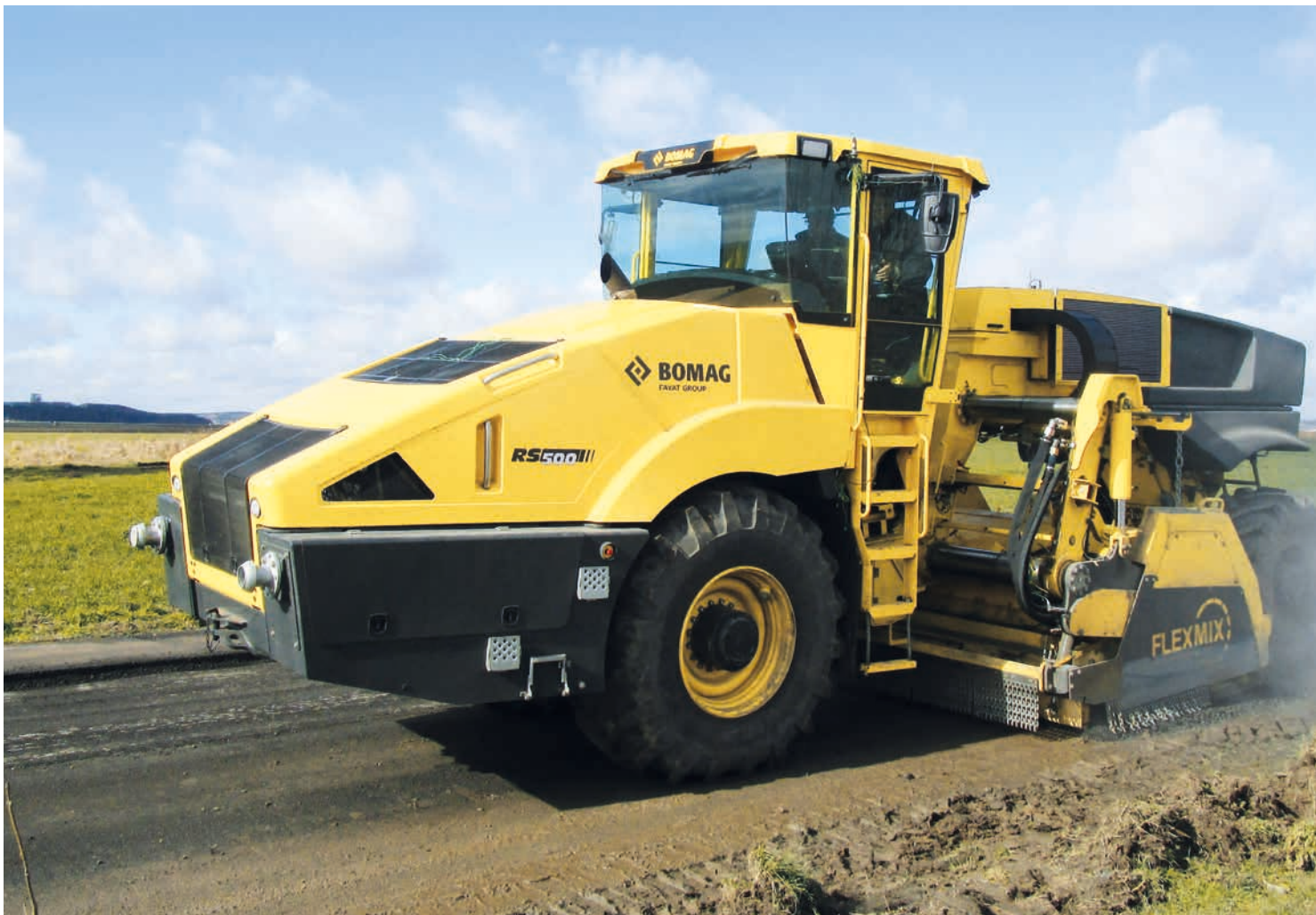
Milling 8 cm of asphalt road.
