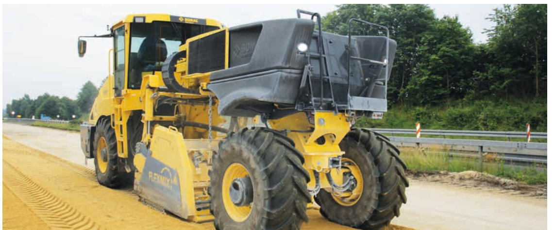
Milling a hydraulically bound base course.
