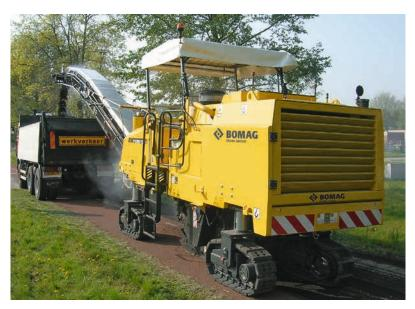
Removal of wear, binder and bearing courses in one pass in sewer construction.
