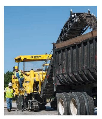
For pavement repairs on country roads the damaged layers are selectively removed. Highly visible marks on the side plates make precise incutting easy.
